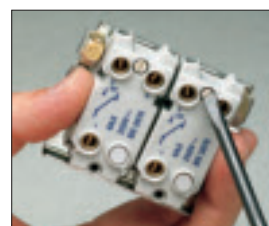
3 Fix switches into grid.
