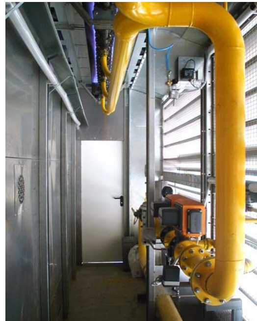
Direct air heating with NP- III AIRFLO® burners in continuous flow dryers for grain.
