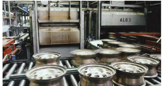
Aluminium age-hardening furnace with air/gas ratio controls for air deficiency cut-out
