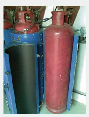
Compressed gas is used during the commissioning and start-up phases of gas turbines, it's critical that a reliable and constant gas supply is available. ISOPAD Hazardous area gas bottle heaters were recently used to guarantee the bottled gas supply met the client's requirements during the start-up ignition sequence at a new plant in Yemen.
