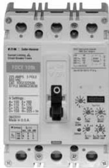
F-Frame Breaker with Electronic Trip Unit
